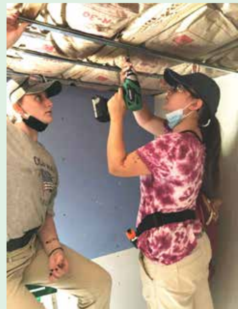
Putting up a ceiling in Kentucky.
