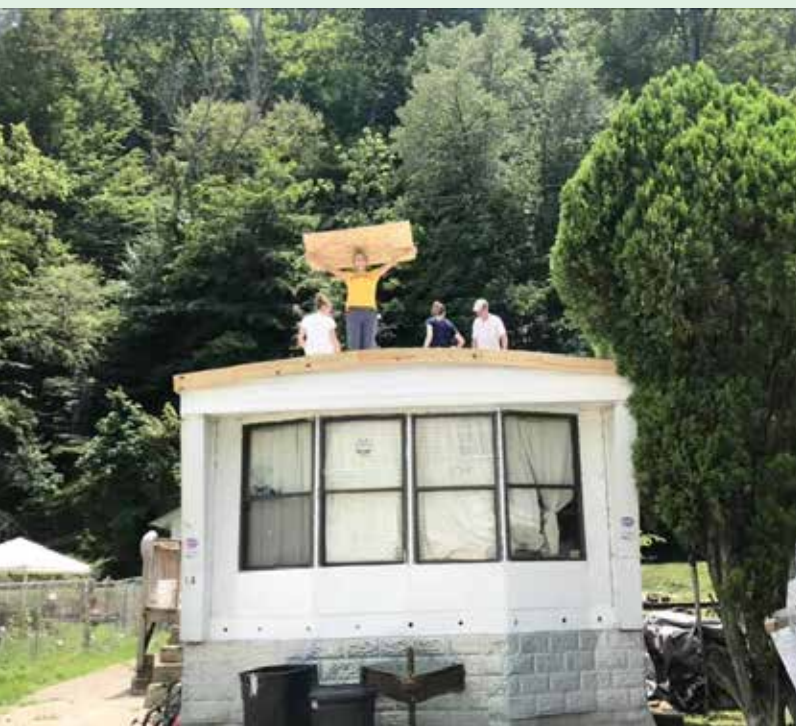
Repairing the roof of a mobile home in Appalachia
